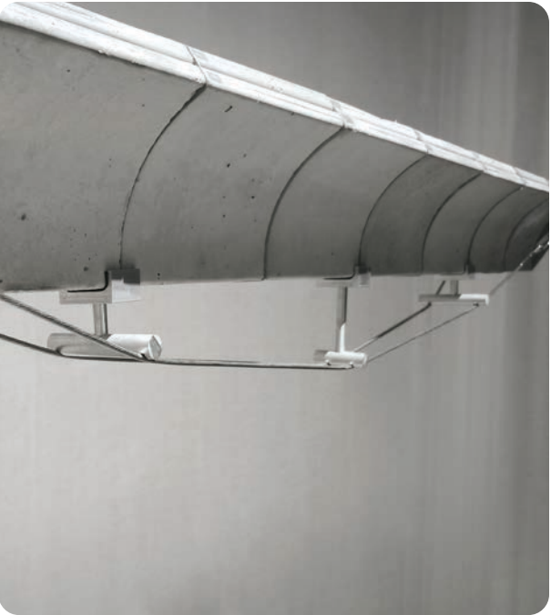
Steel tie rods on concrete bridge
